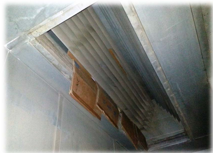
Outside air dampers found to be non-functional and using cardboard to hold outside air back.
